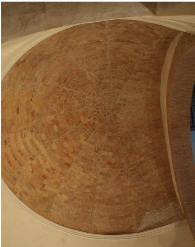
**Fig. 6:** Contemporary brick vault covering the counterapse of Mazote. Remains of the early medieval vault may be observed in the lower part of the image
