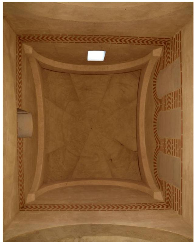
**Fig. 7:** Contemporary vault covering the crossing space in San Cebrián de Mazote
