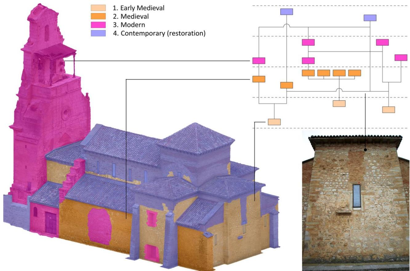
Fig. 15: 3D model of the church of San Cebrián de Mazote with implemented paradata
