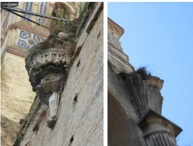
**Fig. 8:** Left: corbel in the choir loft; right: tas-de-charge over one of the pilaster capitals
