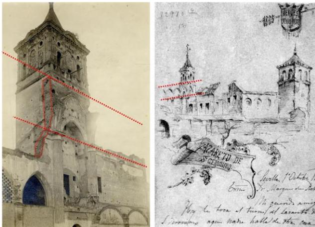
**Fig. 15:** Left: photograph by Nadin showing the wall interface (Fototeca de la Universidad de Sevilla); Right: drawing by Gumersindo Díaz (Sancho 1975)
