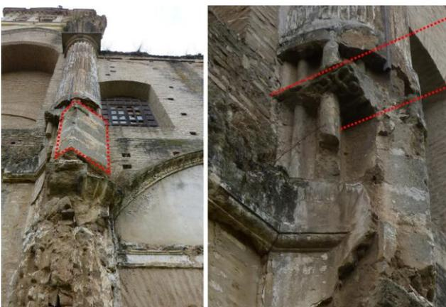
**Fig. 9:** Joint between the mouldings on the choir front and the vault with the pilaster
