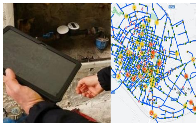
Fig. 9: left , Noise Logger; right , Leak detection via noise loggers in a water distribution network
