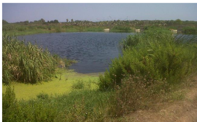
Fig. 2: Constructed wetland as part of the wastewater treatment in Melendugno, Apulia, Italy
