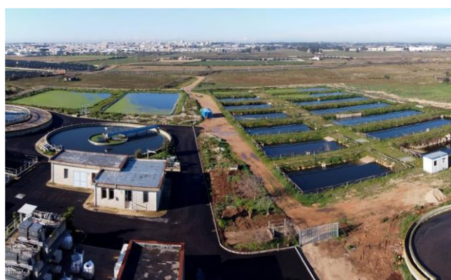
Fig. 5: Wastewater treatment plant with drainage trenches in Galatina, Apulia, Italy
