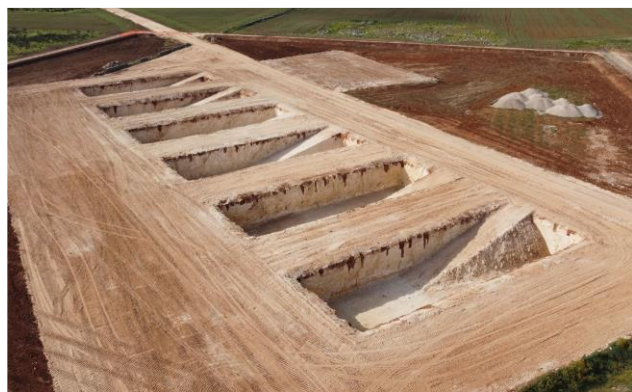
Fig. 4: Newly built drainage trenches in San Cesario, Apulia
