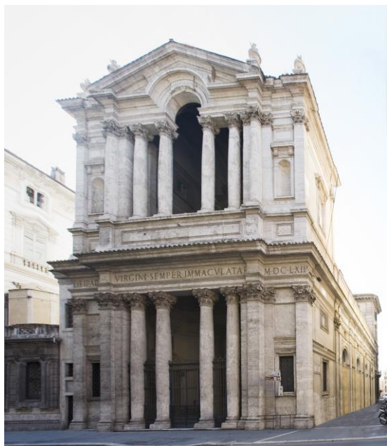
Fig. 1: View of the facade of Santa Maria in Via Lata. Source: ACAS3D Soluzioni Digitali Srl (2010)
