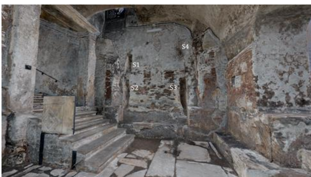
Fig. 7: 3D scanning model of the East Wall in Room II of the crypt of Santa Maria in Via Lata. Highlighted, the four cavity traces identified S1, S2, S3 e S4 (elaboration by ZS).
